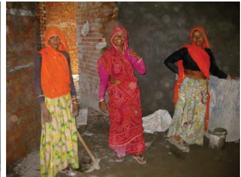
Local ladies employed in construction of girls' shelter home
