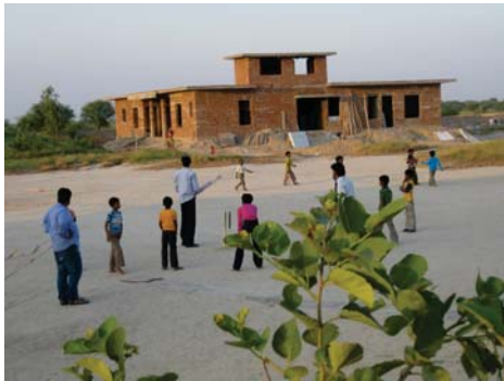
Girls' shelter home under construction in background
